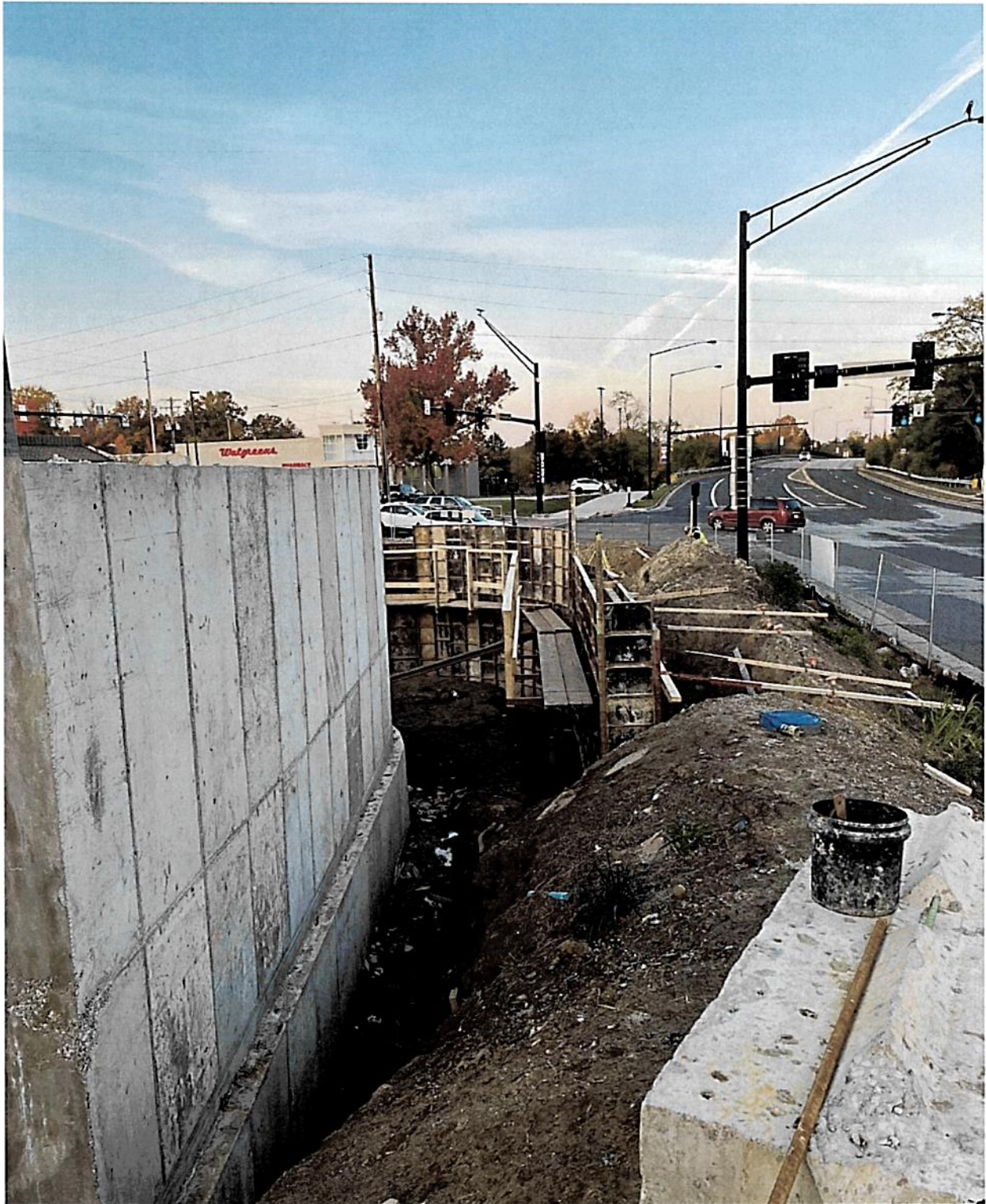
North Side Haymaker Parkway Side Retaining Walls
