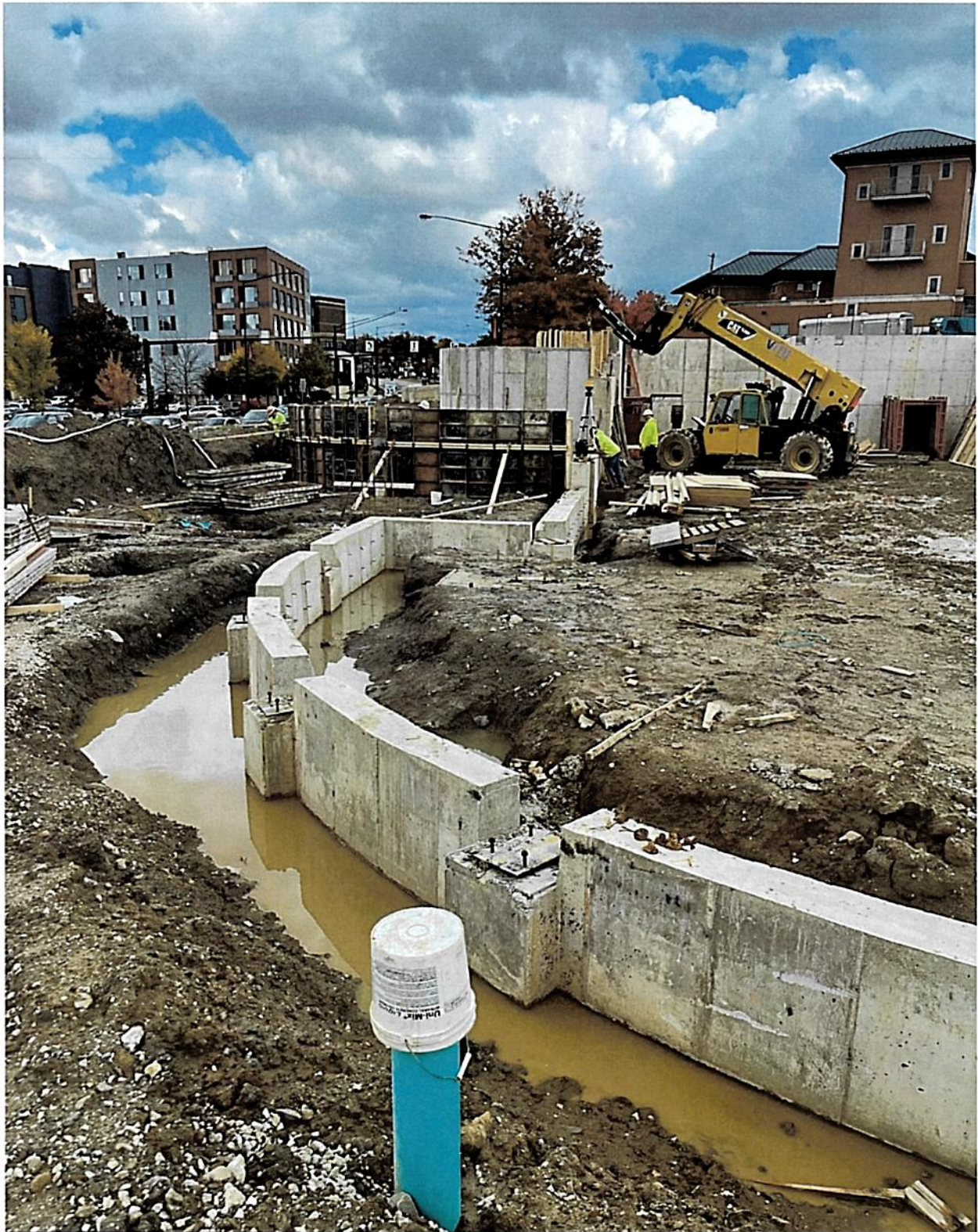
Front of Atrium S. Water Street and Haymaker
