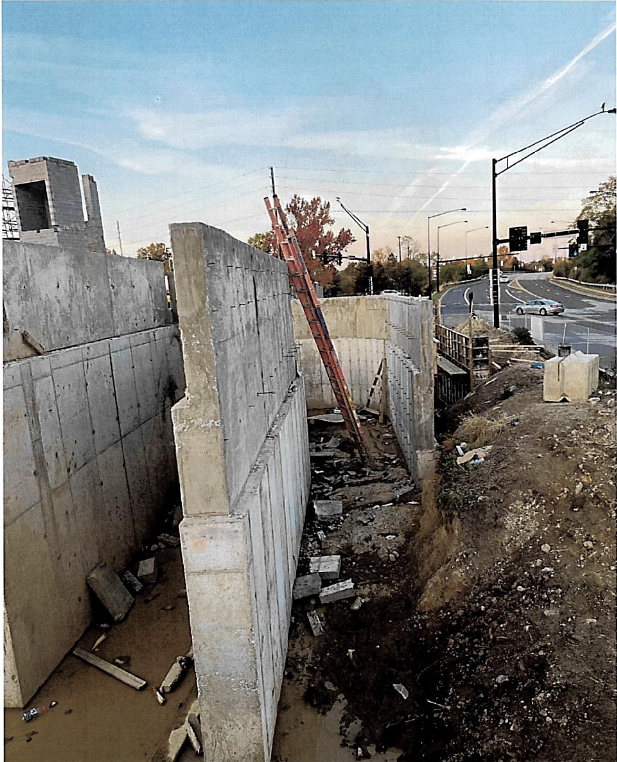
North Side Haymaker Parkway Side Retaining Walls
