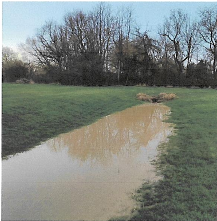
Picture #6 – Another Picture Showing the “river” that forms after rainfall Flowing into a culvert
