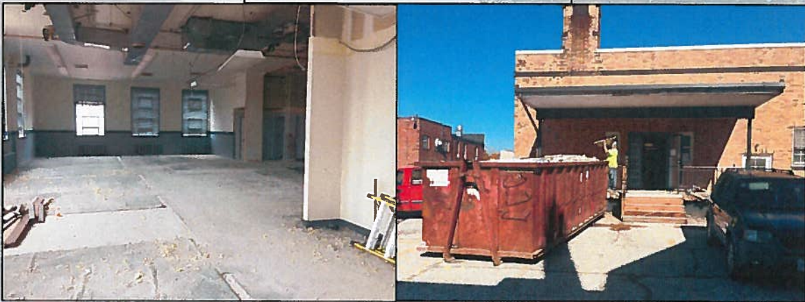
John Flynn Courthouse Renovation
