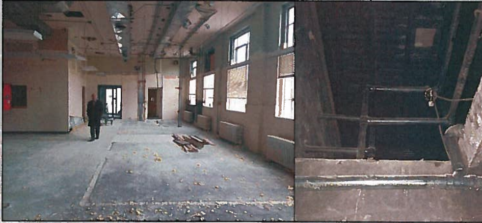
John Flynn Courthouse Renovation
