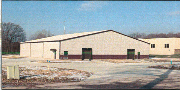
Enterprise Plastics New Warehouse
