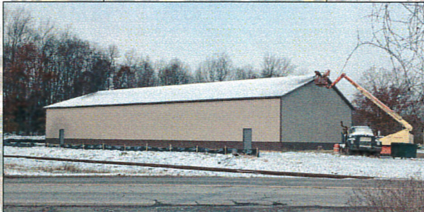
Allen Drain Service New Warehouse
